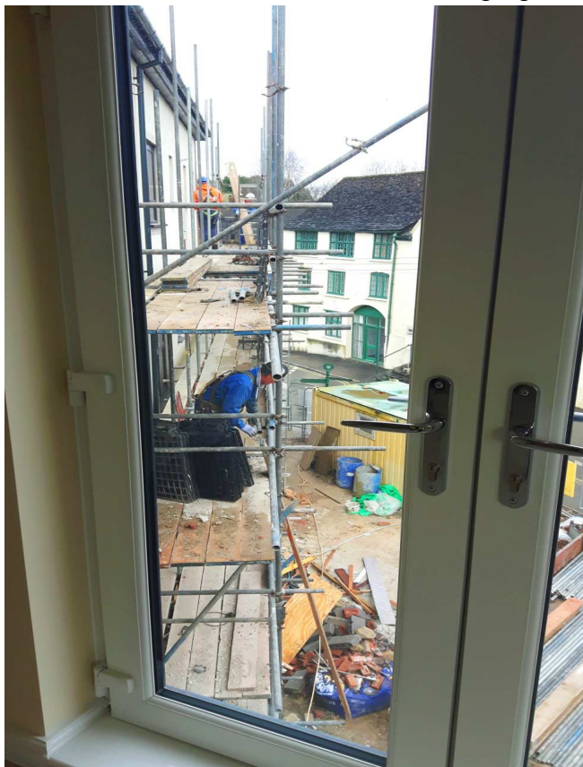
Affordable flats under construction in Dursley, 2017
