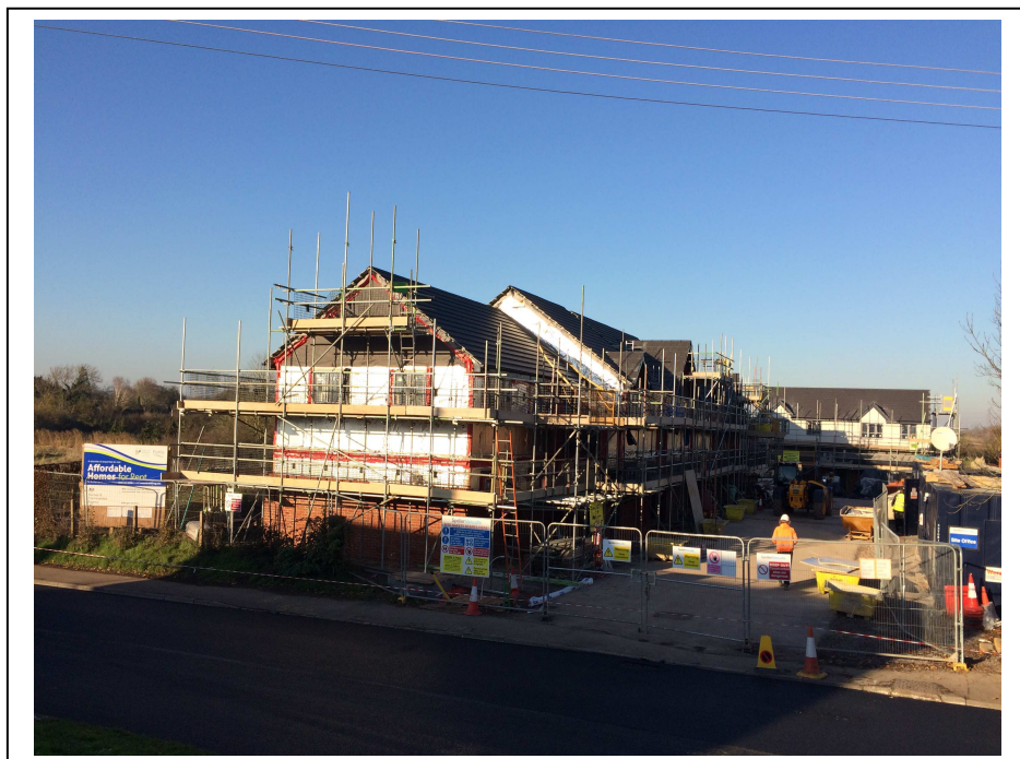
Lynch Road, Berkeley Rural Exception site under construction 2016
